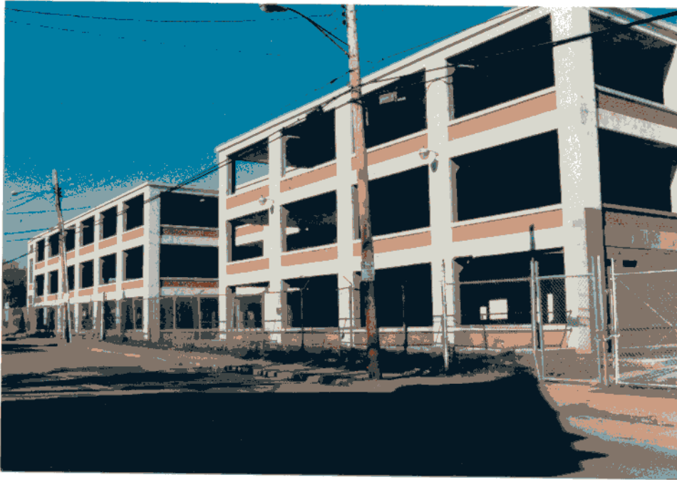
Veeder Place at the northern border of Asylum Hill is currently undergoing rehabilitation.
