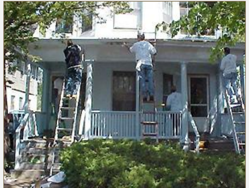
Rebuilding Together Hartford Volunteers repair a home
