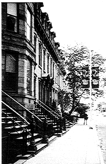
The brownstones along Capitol Avenue
