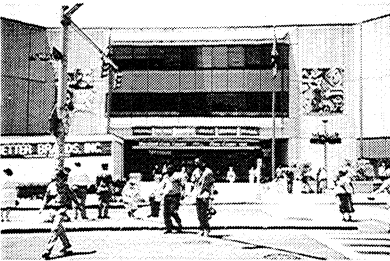
The Hartford Civic Center will soon be renovated.
