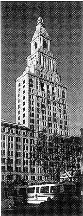
The Traveler's Building recalls an earlier era of sophisticated urban architecture
